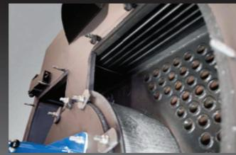
The CRG stack economizer acts as a waste heat recovery device, ensuring that this available heat does not go unused. Instead, the heat is recovered to essentially preheat the boiler's makeup water.
